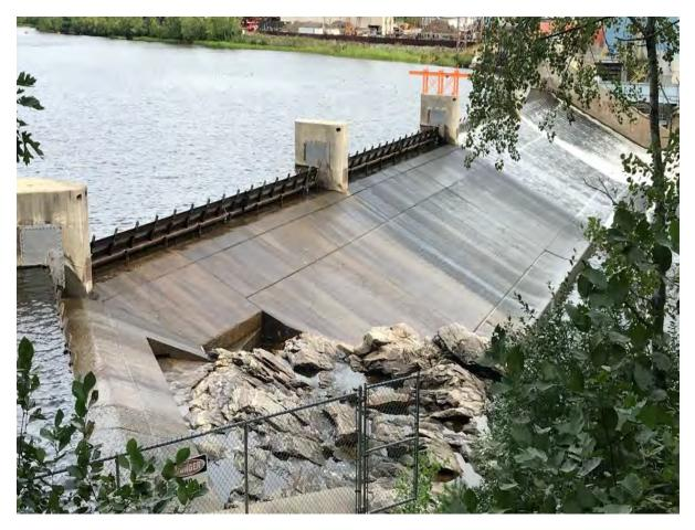
Figure 5.0-4: Exposed Bedrock Area Below Bascule Gate No. 5 (10:31 am)
